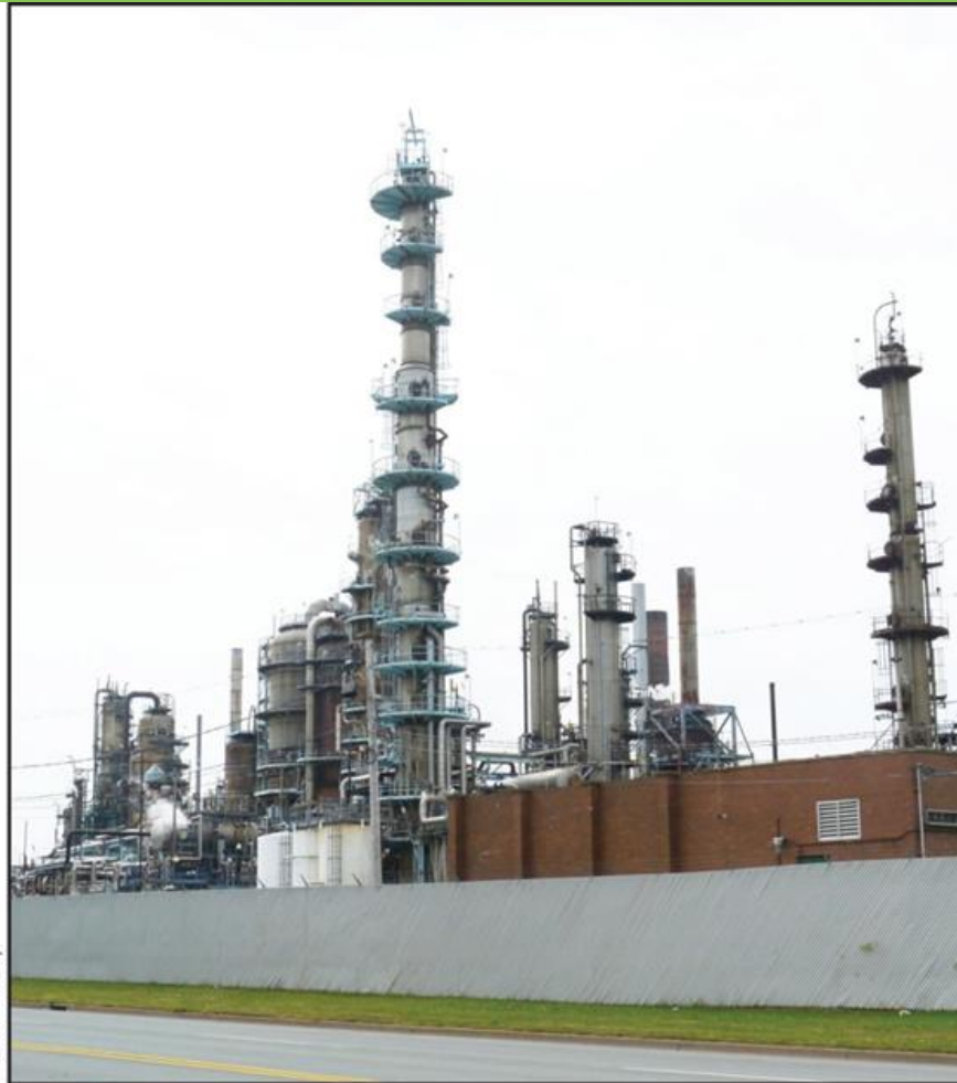
Figure 3.8: Fractionating columns at Dartmouth Refinery, Dartmouth, Nova Scotia.
